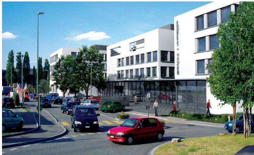
The new headquarters of the Endress+Hauser Group in Reinach (from late 2006).
