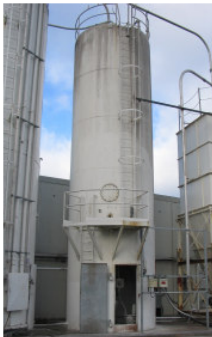
The 30 tonne skirted Flour Silo
