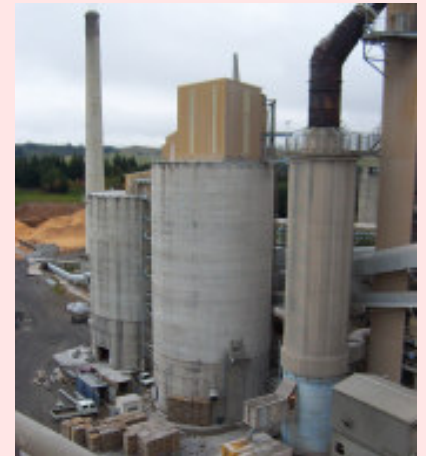
Golden Bay Cement Silos
