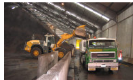
Loading the truck in coal storage building prior to weighbridge checking
