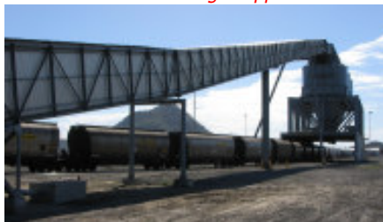
Enclosed coal load-out conveyor system. Picture below shows a train being loaded from the storage hoppers.
