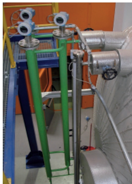
Levelflex M on feedwater container
