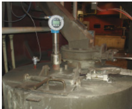
FMP45 Guided Radar on Coal Reject Hopper
