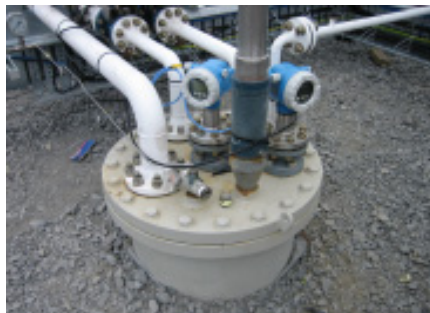
FMP40 Guided Radars on LPG Bullet Tank
