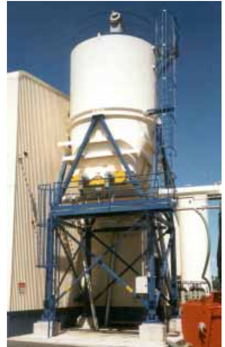
Wastewater Treatment Plant Sludge Tank
