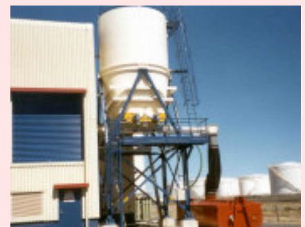
EMC Vessel Weighing installation with DSM Loadcell Mounts
