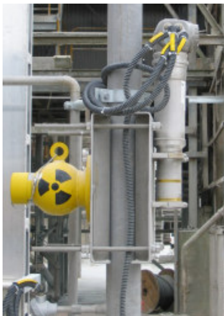
Source Container and Gammapiilot M FMG60
