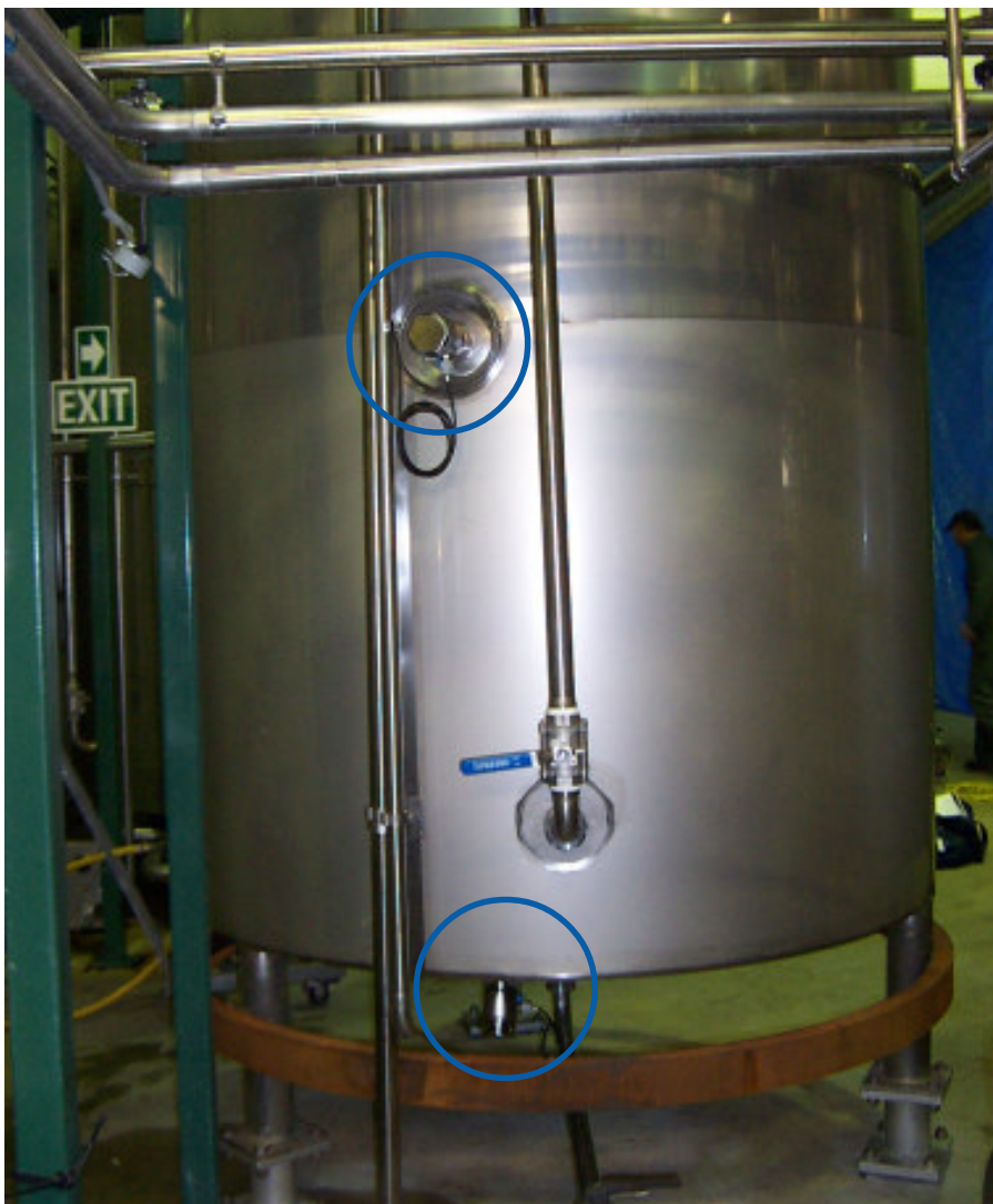
Batching Tank at Frucor Beverages Ltd with 2 Deltapilot S Pressure Transmitters (circled)
